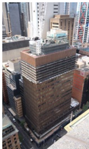
Upgrades begin at 20 Martin Place. Photo: Built
